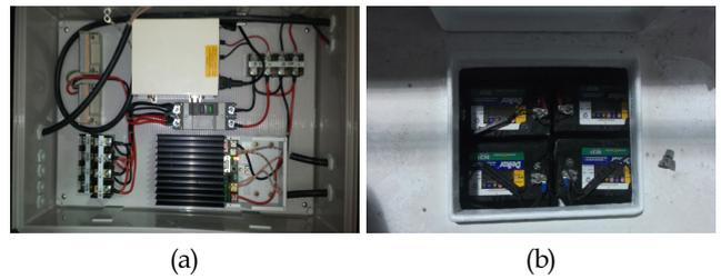
Fig. 15 The view of charging inverter component (a), battery for supplying electro-motive force (b)
